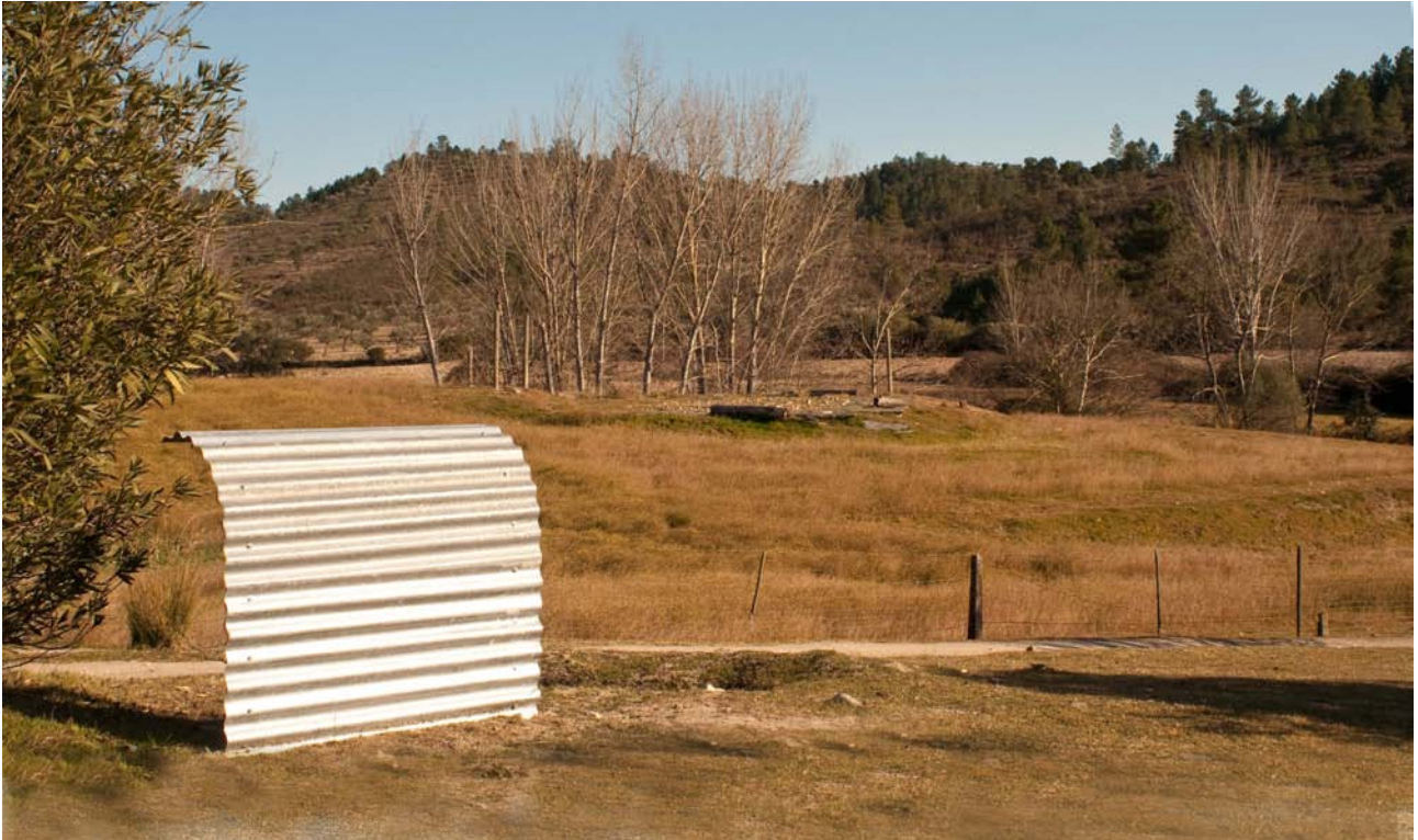
Guard for the water meter
